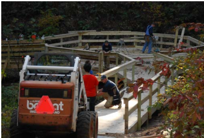
Volunteers put the finishing touches on the end of the boardwalk.
