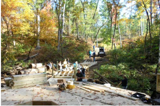
Volunteers work on the observation platform, which has a fire pit.
